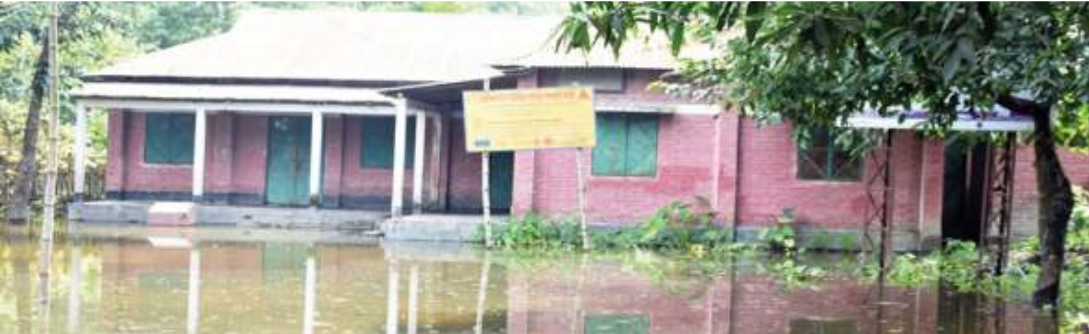
An NGO office in flood-prone area of Moghulbasha
